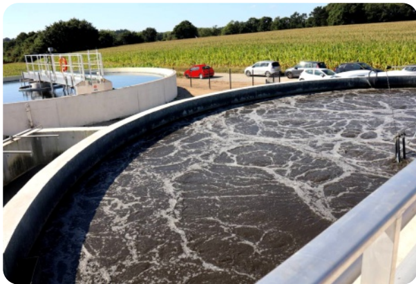
Dissolved oxygen measurement in aeration tank
